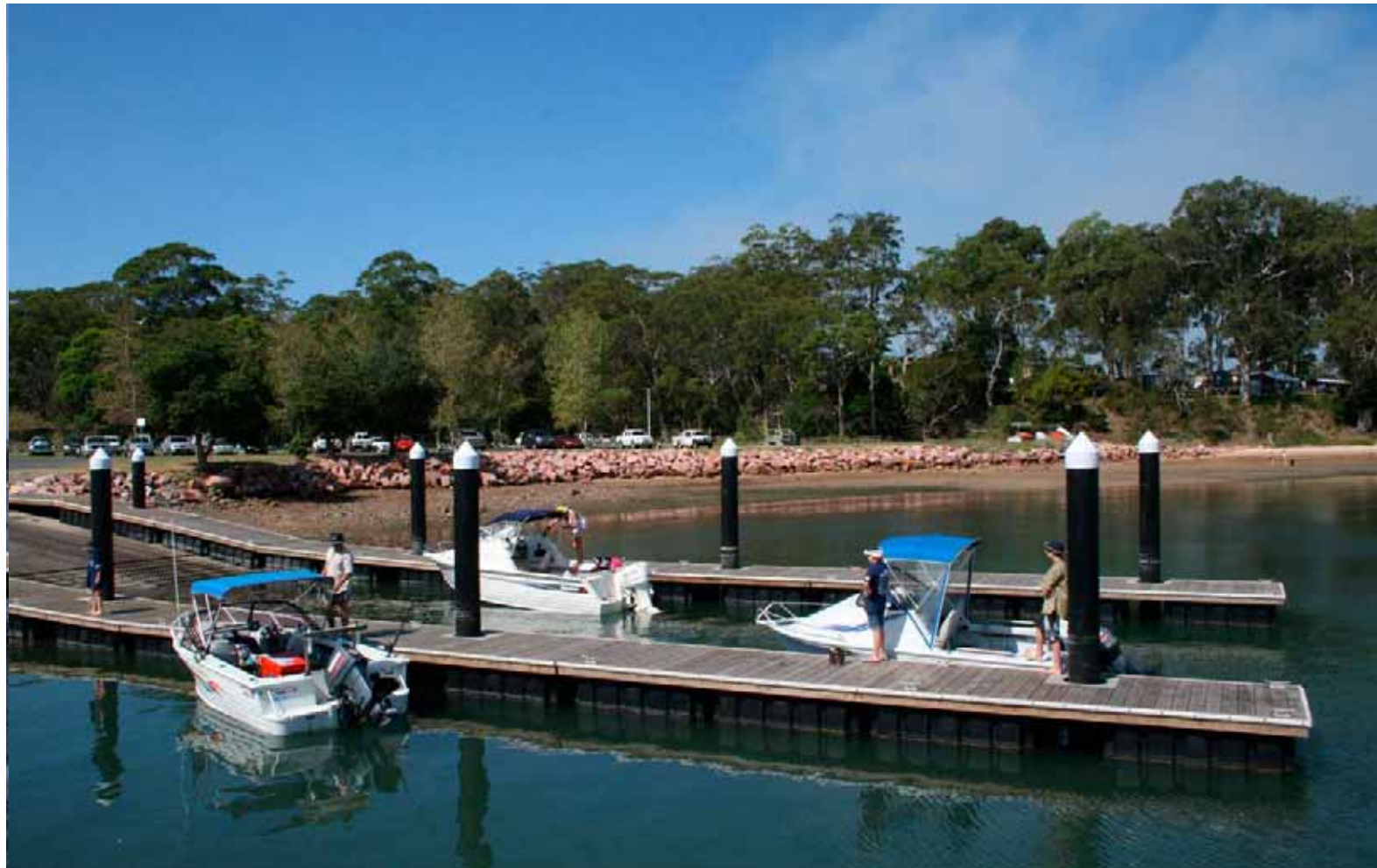
Widening of boat ramp to three lanes and installation of two modular on-ramp pontoons.
