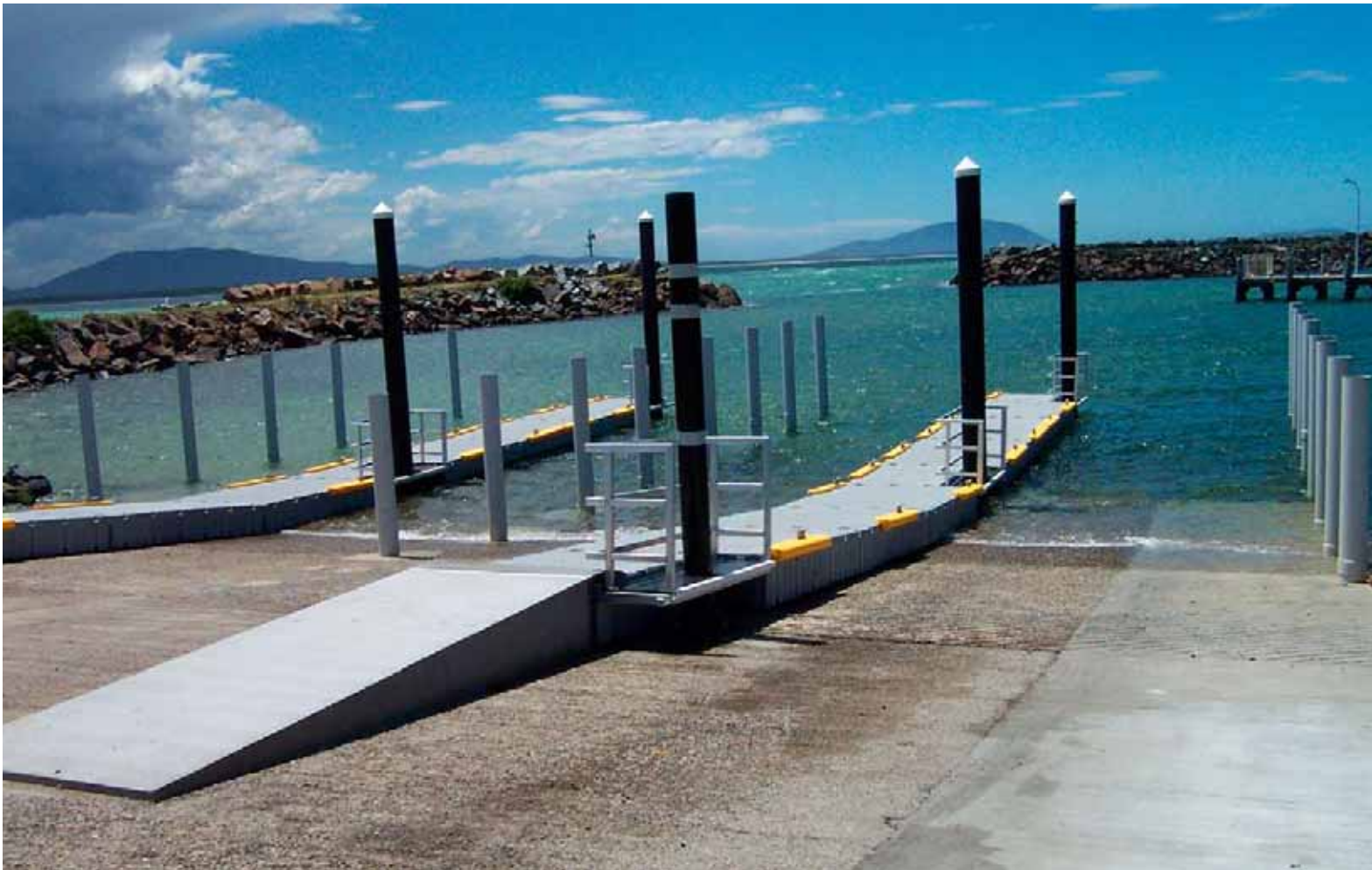
Removal of landing platforms, widening of boat ramp, provision of pontoon access and provision of surge poles (to assist with launching and retrieval).
